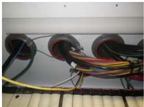
WIRING IN PLC CABINET SHOWS MULTIPLE GROUND BONDS
