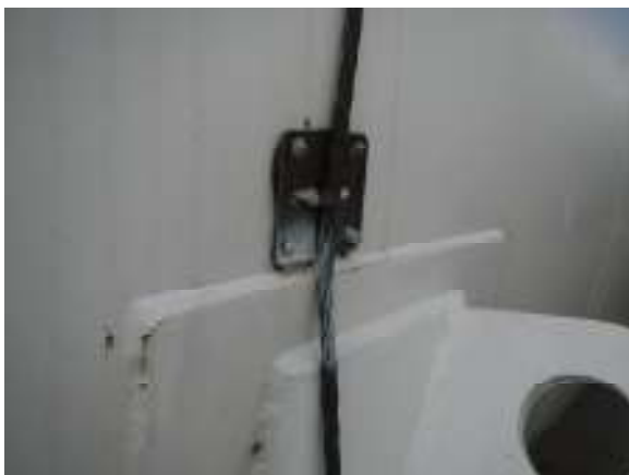
UN-GROUNDED STATIC TIE WIRE, TANK NOT BONDED
