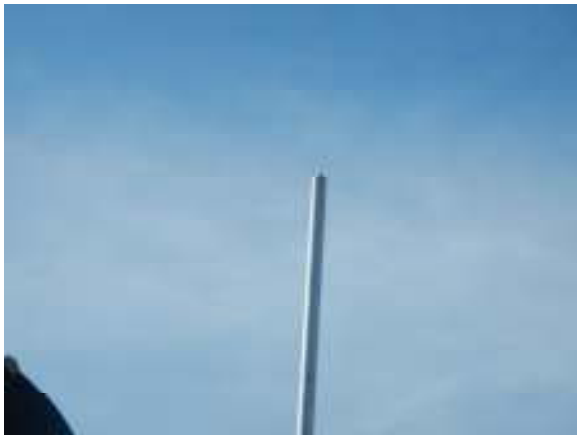
DEFECTIVE STATIC TERMINAL, ROUNDED NOT EVEN BEVELED
