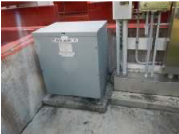
UN-GROUNDED TRANSFORMER WITH NO TVSS
