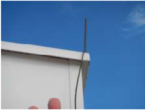
DEFECTIVE ROUNDED STATIC ROD
