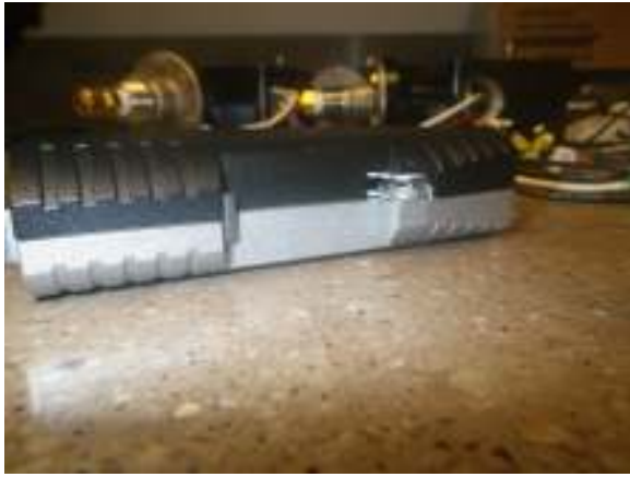
EXAMPLE OF SYSTEM WIDE CAT 5-6 LAN SURGE TVSS, REQUIRES FULLY GROUNDED DIN RAILS
