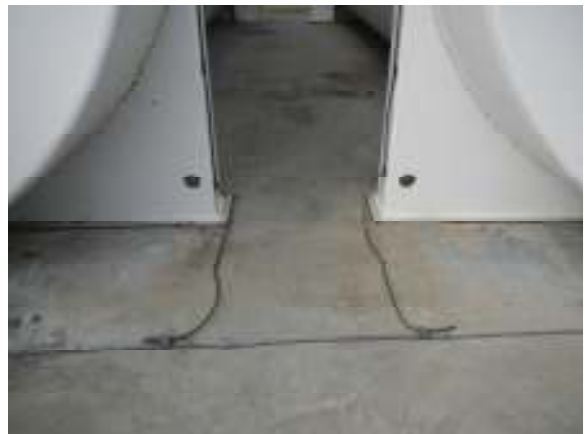
DIESEL TANKS, STATIC RODS, TANKS NOT DIRECT GROUNDED. GROUND ONLY THROUGH PIPING
