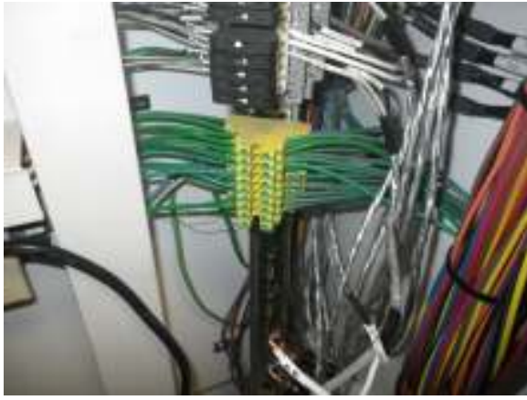
EXAMPLE OF GROUND STAR IN PLC CABINET. THIS SHOULD BE REPEATED IN ALL CABINETS
