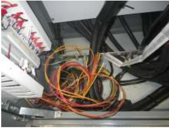
INSIDE OF HSPS VFD, ARC AND SHOCK HAZARD, UN-TERMINATED WIRES, POOR SERVING
