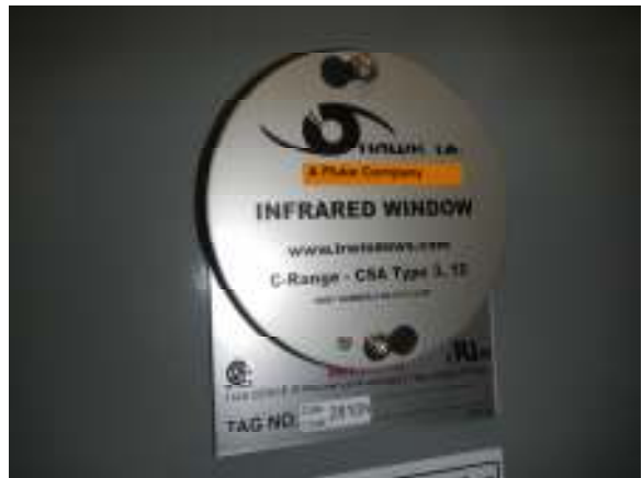
INFRA RED SURVEY PORTAL ON MAINS DISCONNECTS
