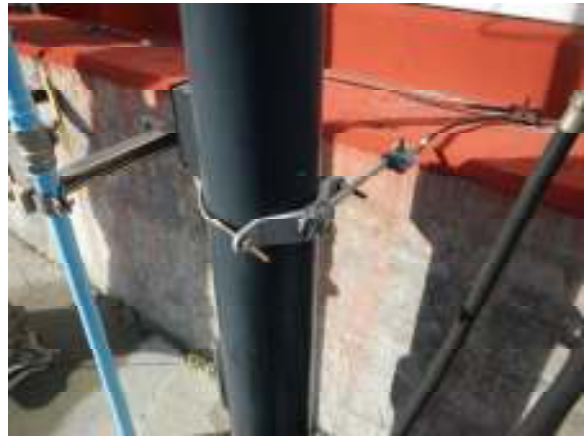
POOR GROUND ON STREET LIGHT
