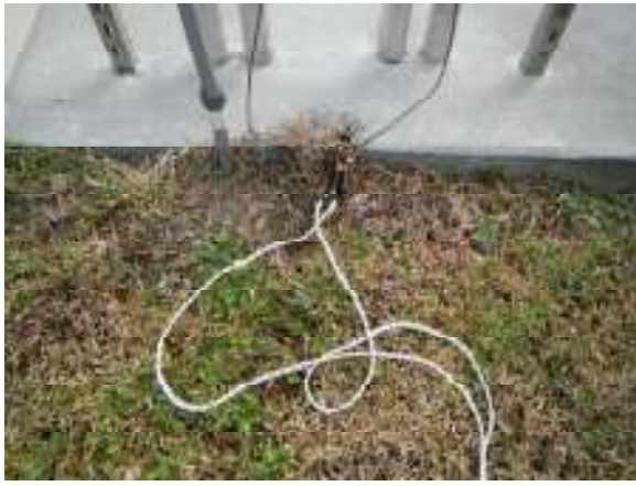
FPL METER CAN GROUND SYSTEM., 1 OF 2, SHALLOW ROD, POOR OHMIC VALUE
