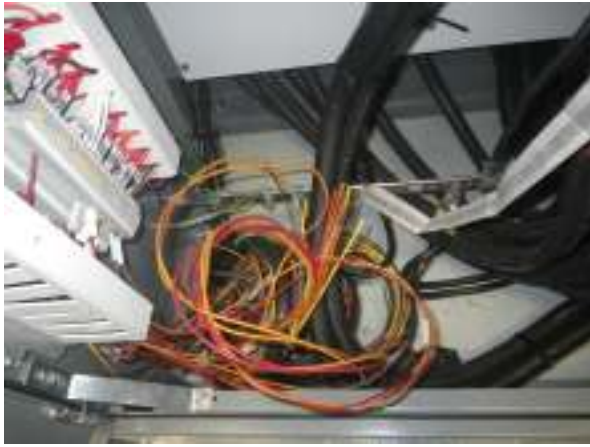
Example of hazardous wiring
