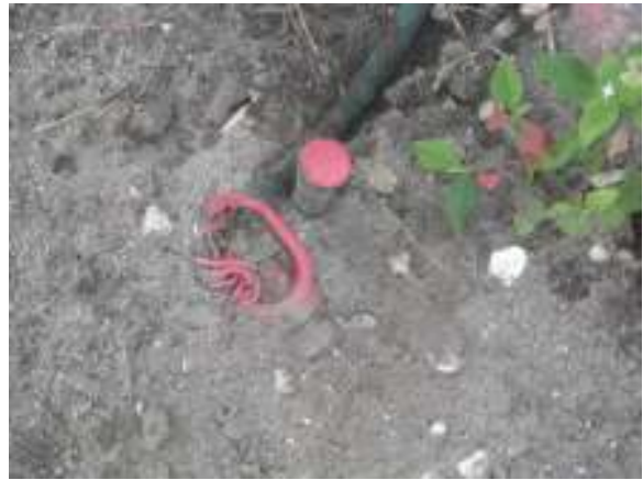
BROKEN GROUND CLAMP AT HSPS GENERATOR
