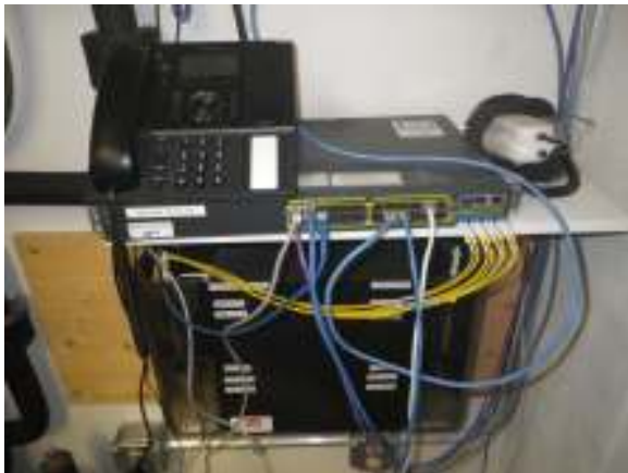
NO SURGE TVSS ON LAN FEEDERS TO PROTECT FIBER SWITCH
