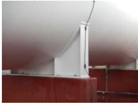
TANK NOT GROUNDED, STATIC WIRE NOT ATTACHED TO TANK
