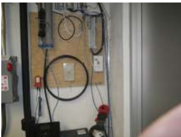
SINGLE END GROUND ROD IN TELEPHONE SHELF, POOR OHMIC VALUE
