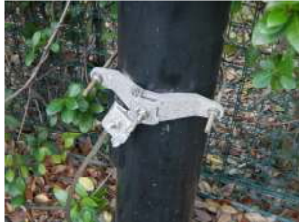
How not to connect a lamp post to earth.
