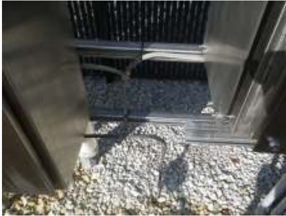
PROPERLY CADWELDED GROUND CONNECTIONS WELL HR6
