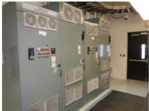
BLOWER ROOM, CONCENTRATOR VFD
