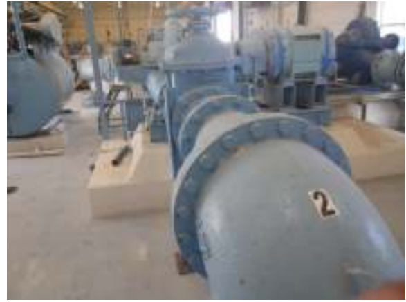
HSPS PUMP 2, BAD OUTBOARD BEARING AND CLOGGED AIR FILTERS, MOTOR TEMP 212+
