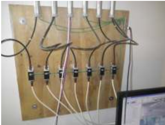
CAMERA TVSS PANEL IS NOT BONDED TO A REAL ELECTRICAL GROUND AND RELIES ON COAX CONNECTIONS TO UNKNOWN LOCATION
