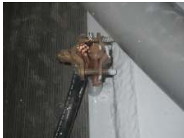
Improper ground connector as seen in multiple locations
