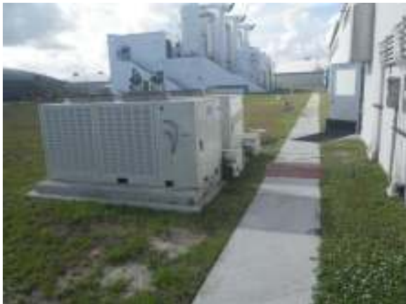
AIR CONDITIONERS, HSPS ELECTRICAL ROOM
