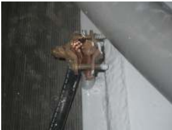
SINGLE END GROUND ROD, 1 OF ONLY 6 ON SITE
