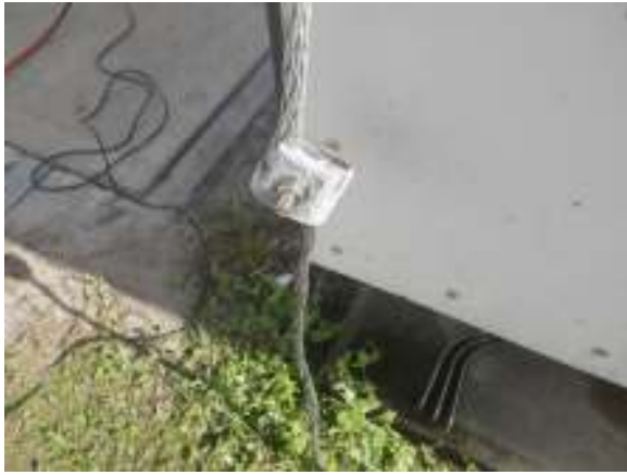
CORRODING STATIC ARRAY SPLICE
