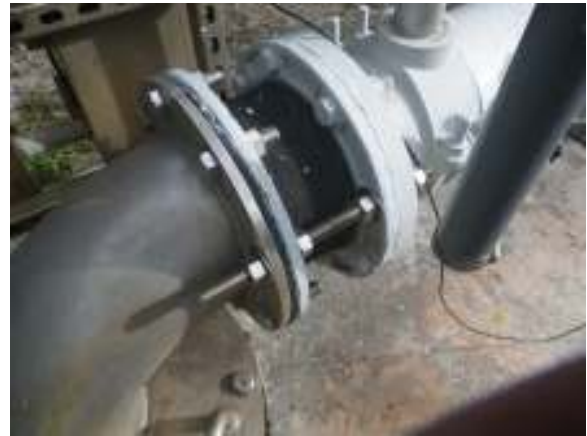
MOTOR SLEEVING AND DISCHARGE PIPING NOT WELL BONDED
