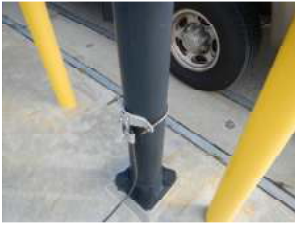
EXAMPLE OF NUMEROUS LIGHTING POLES NOT WELL GROUNDED THROUGH PAINT
