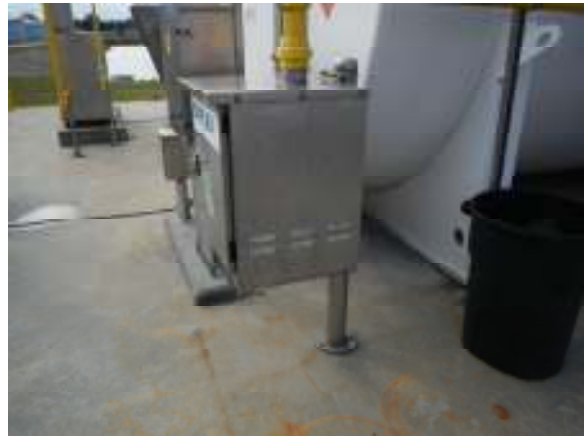
DIESEL FILL PORTAL NOT GROUNDED
