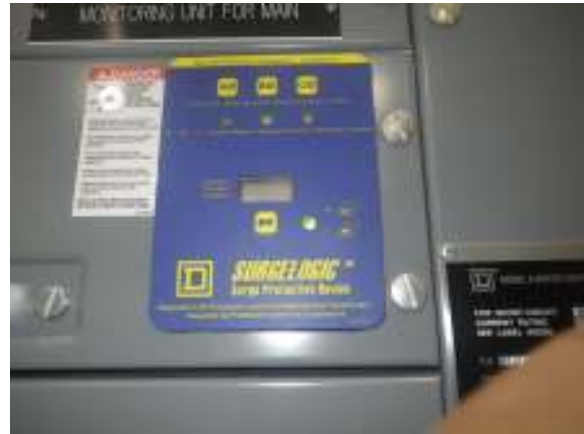
EXAMPLE OF EMBEDDED TVSS IN MAINS ROOM, MCC 1, 2
