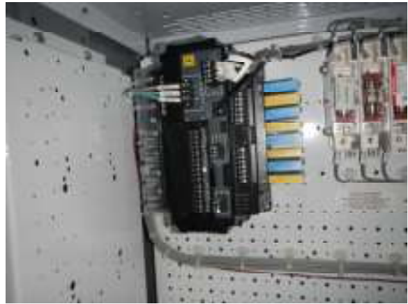
POWER MONITOR SYSTEM SQUARE D NEEDS MOD BUS TO LAN CARDS ORDERED AND INSTALLED WITH SOFTWARE
