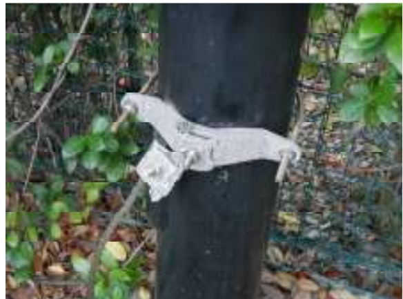
POOR GROUND CONNECTION
