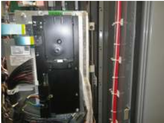
ROCKWELL TECHNICIAN INSTALLED A STATIC STRAP ON A FULLY GROUNDED CHASSIS FOR AN UNKNOWN REASON
