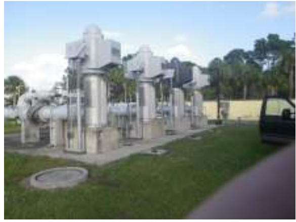
TRANSFER PUMP ROW, NEEDS OVER BRIDGE STATIC LINE
