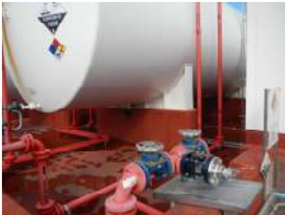
CHEMICAL TANKS NOT PROPERLY GROUNDED
