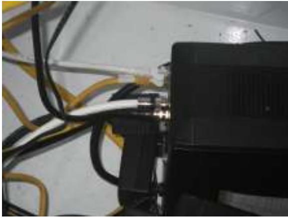
COMCAST CABLE FEEDER GROUNDED THROUGH UPS. UPS DOES NOT HAVE A DEDICATED GROUND, ONLY THROUGH PLUG
