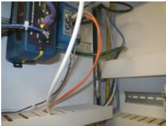
MICROWAVE COAX TVSS WITH POOR GROUND CONNECTION AND NO TVSS AT ENTRY POINT TO BUILDING
