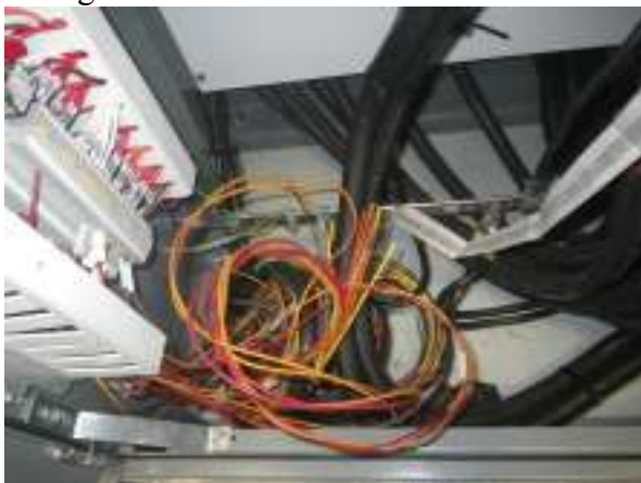
Example of hazardous wiring
