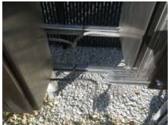
PROPERLY CADWELDED GROUND CONNECTIONS WELL HR6
