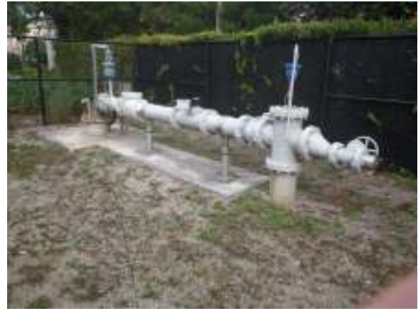
WELL EXAMPLE OF SUBMERGED DRIVE
