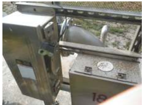
MOTOR SLEEVING AND DISCHARGE PIPING NOT WELL BONDED
