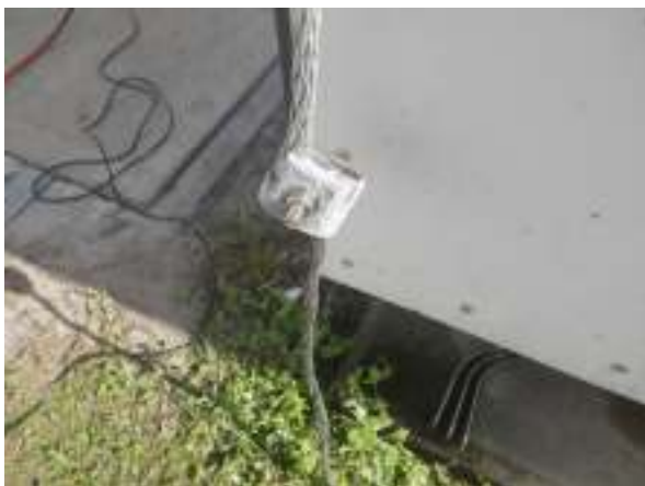
Example of badly corroded joiner
