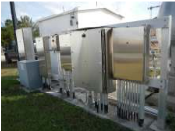
INJECTION WELL ELECTRICAL PANELS
