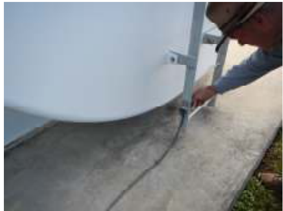
TANK INDIRECTLY GROUNDED THROUGH DISSIMILAR METALS LADDER ATTACHMENT
