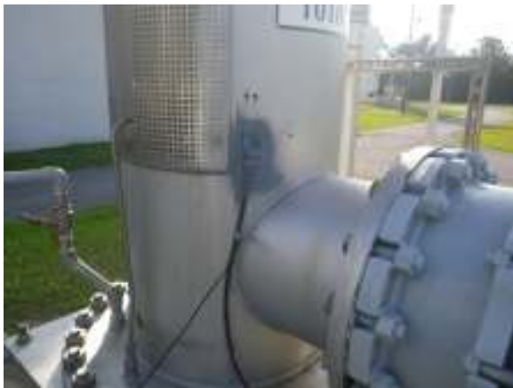
BROKEN STATIC TERMINAL CONNECTION PUMP 1 AND 4 OF TRANSFER PUMPS.
