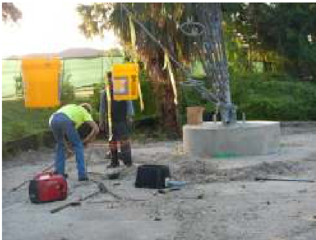
Note meter box, conduit entry point and rods being assembled
