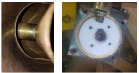
Once the soot was brushed out of the inner TEE on both ends, and chemically cleaned. The freshly cleaned bullets and their dirty deeds were re-torqued and Mr. Burner applied his brute force.
